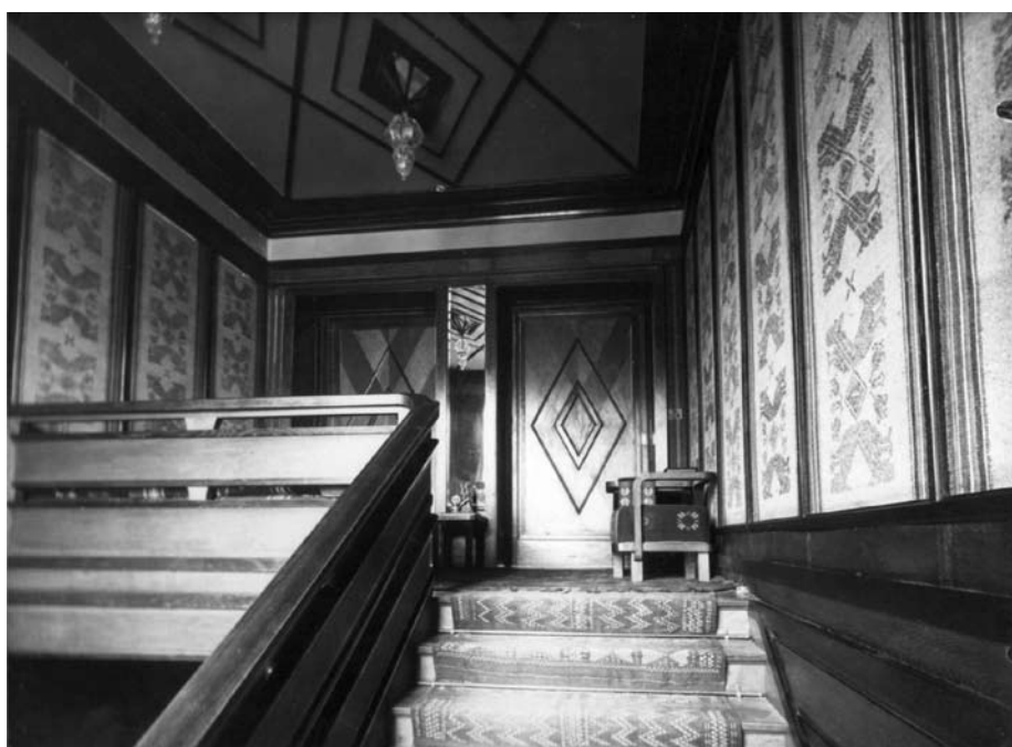
Fig. 21. Vailokaitis' family residence Vieniybės square 8, Kaunas. 4th decade of the 20th century. Corridor of the staircase. Photo from Kaunas Regional Library. I 5715.
