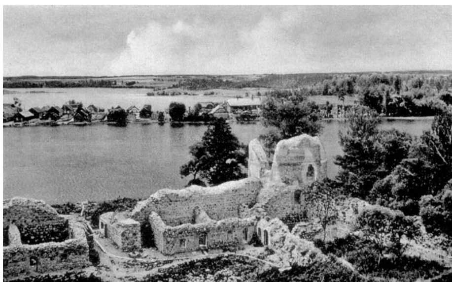
Fig. 6. Interwar building ruins of south-westward forecastle of Trakai Island Castle. Mostly ruined part is western casemates
