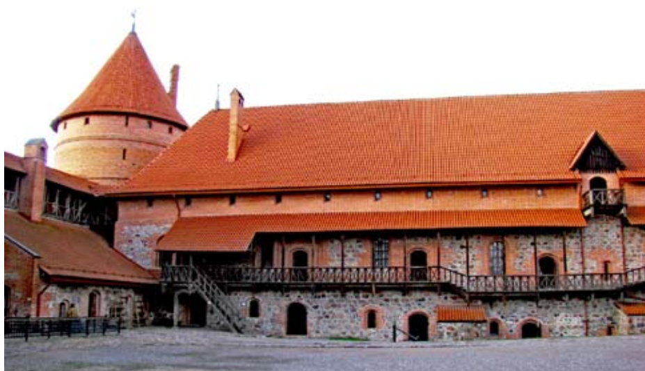
Fig. 7. Reconstructed southern part of the western casemates of Trakai Island Castle
