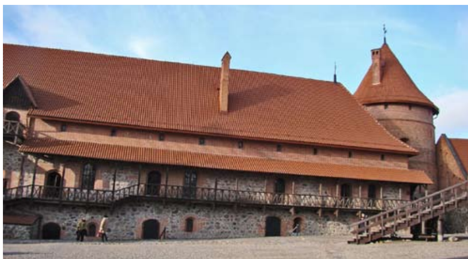
Fig. 8. Reconstructed northern part of the western casemates
