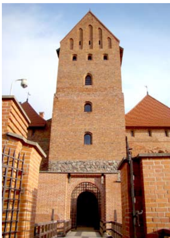
Fig. 4. Reconstructed southern donjon facade of Trakai Island Castle
